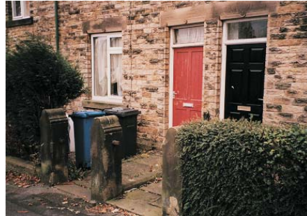
Stone gate piers and stone paving at Nos. 327 and 329 Baslow Road
